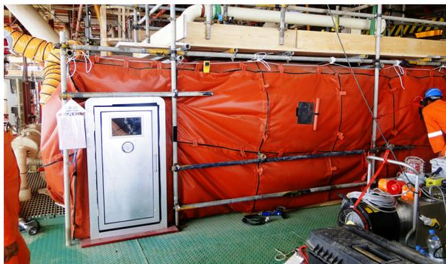
Figure 1. Hot-Hed's Habitat® HWSE deployed on a major offshore platform.
