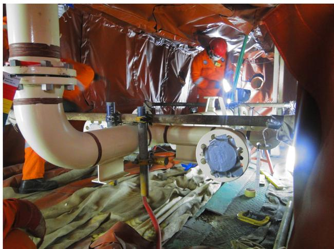
Figure 2. Offshore welding in safety inside a custom configuration of Hot-Hed's Habitat.
